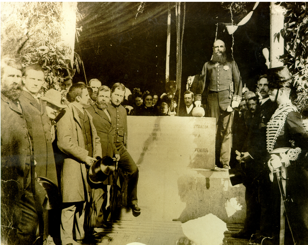
Figure 4: Governor Broome laying the foundation stone of the Victoria Public Library, 1887, (State Library Western Australia, 000617D)
