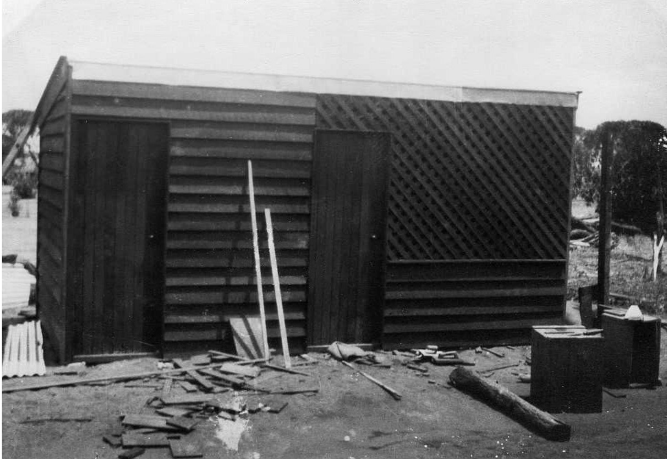
Yealering. A new wash house 1930s, complete with built-in copper & cement troughs, and an adjoining shower room.
