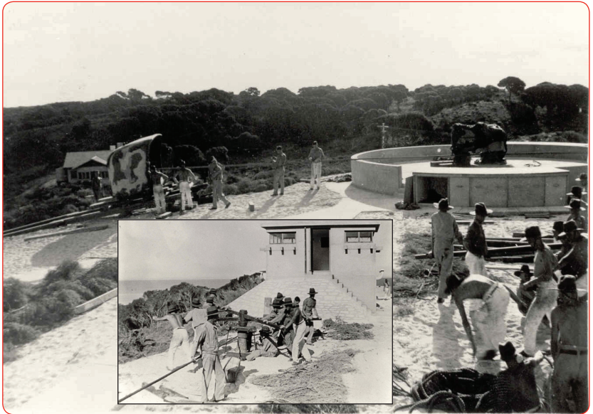
Bickley Point - Hauling the Bickley F2 gun shield onto the gun position after it has been unloaded from the railway trolley. Personnel are using a timber sleigh on rollers that is being hauled up with a grab capstan (just in view on right - see inset).
