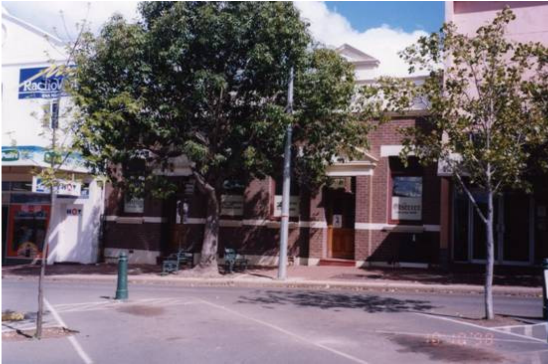
Observer_off Narrogin Observer office (present) Federal Street
