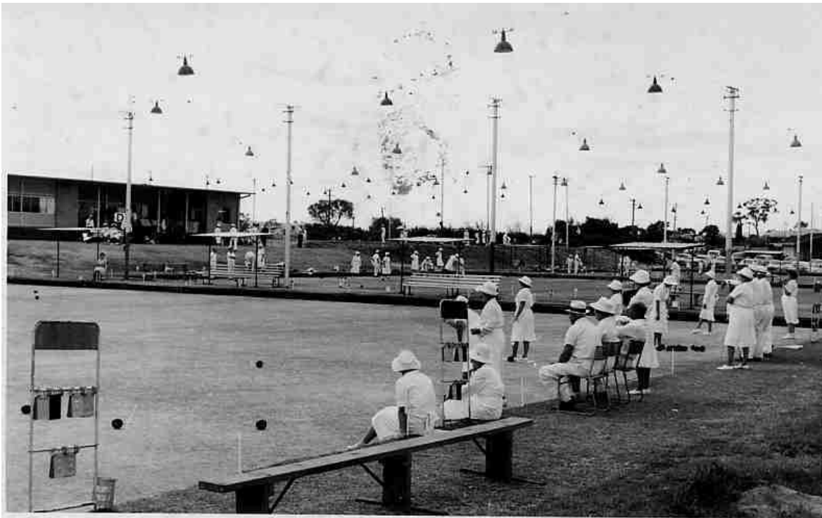
Mixed bowls in Northam before the new seats, shades, lights, brick paving and synthetic greens.
