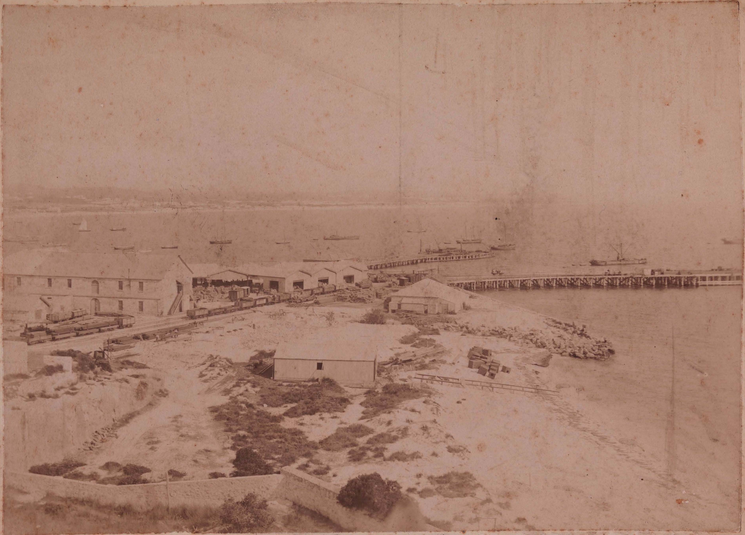
Railway Sheds End of Pier
