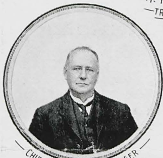
— CHIEF MECHANICAL ENGINEER — — MR. E. A. EVANS —
