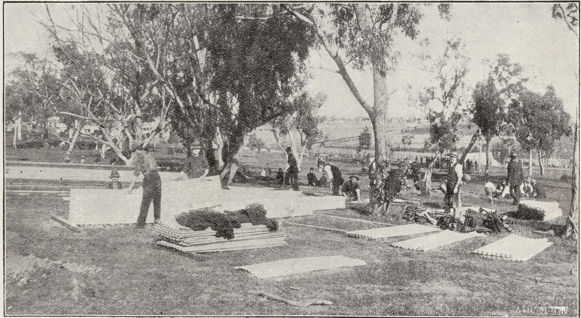
Straightening the iron, of which 2500 sheets were used on the structure.
