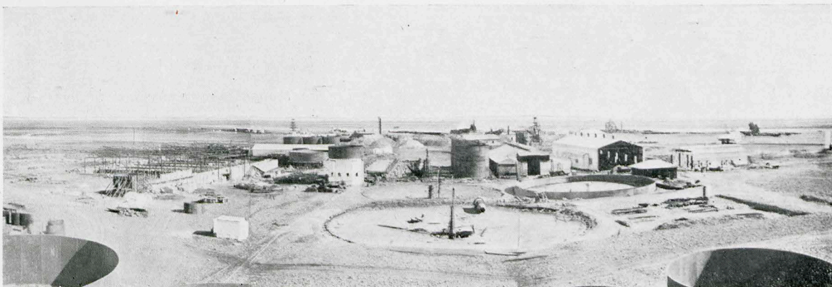
Plant at Wiluna Gold Mine under Construction
