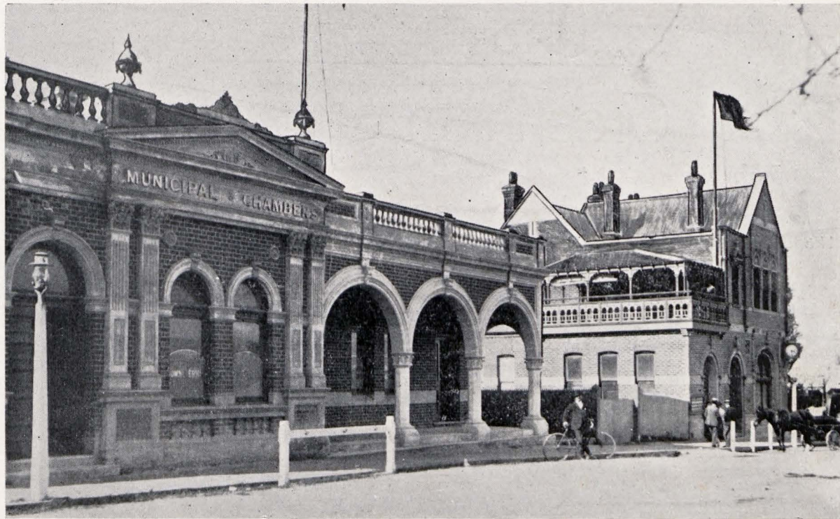
Municipal Buildings and Post Office, Bunbury.
