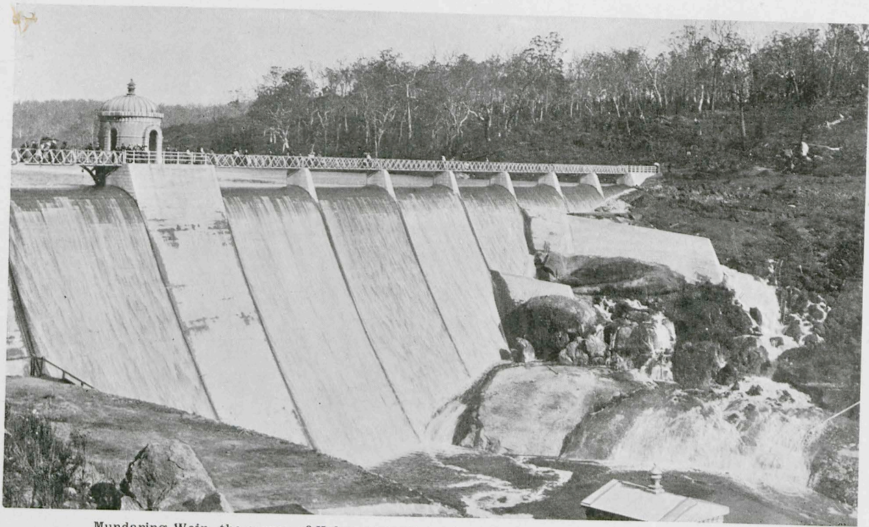
Mundaring Weir, the source of Kalgoorlie's Water Supply. Water pumped from the Weir in the Darling Ranges, a distance of approximately 350 miles.
