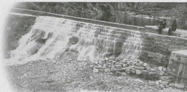
“Saunders’ Weir,” Depot Creek, in the Flinders Ranges (Eastern End).
