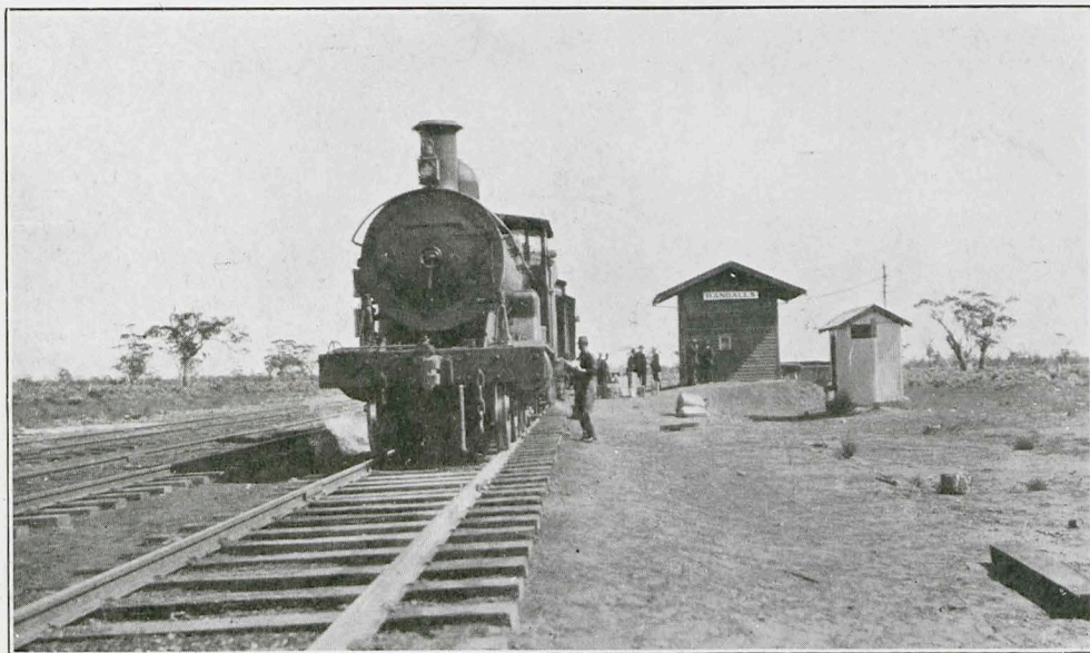
A Typical Roadside Railway Station.
