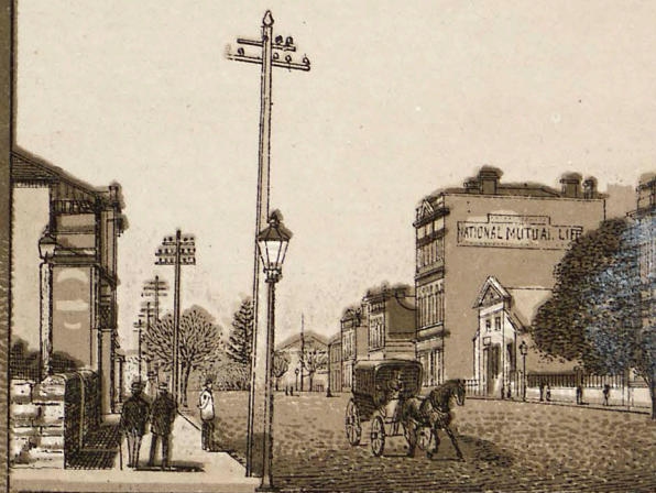
ST. GEORGES TERRACE, LOOKING EAST.
