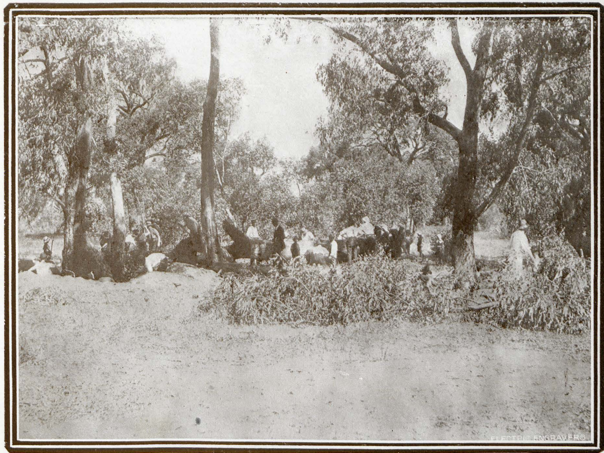
"Busy Bees" Clearing the Site.
