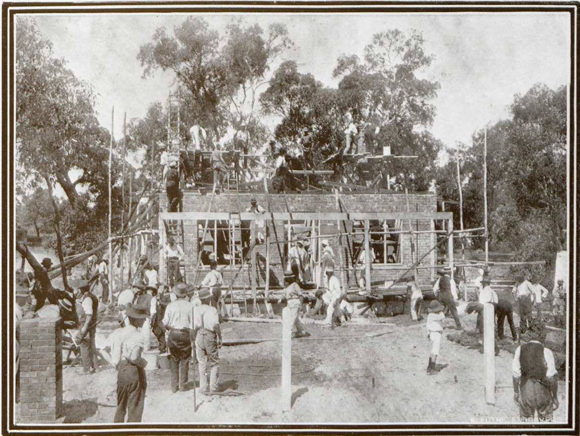
Building Anzac Cottage—Progress made by the "Busy Bees" up to 2 p.m.
